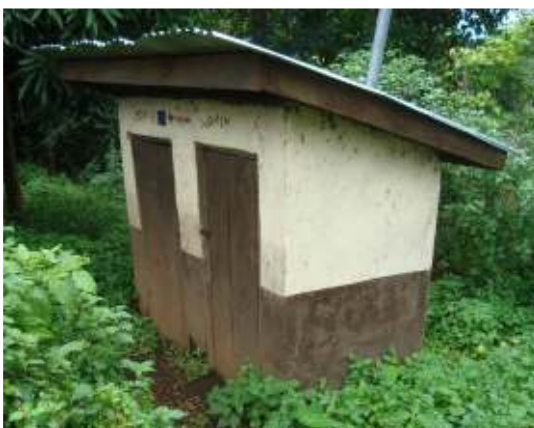
Latrine in Koinadugu district after 2 years of use
