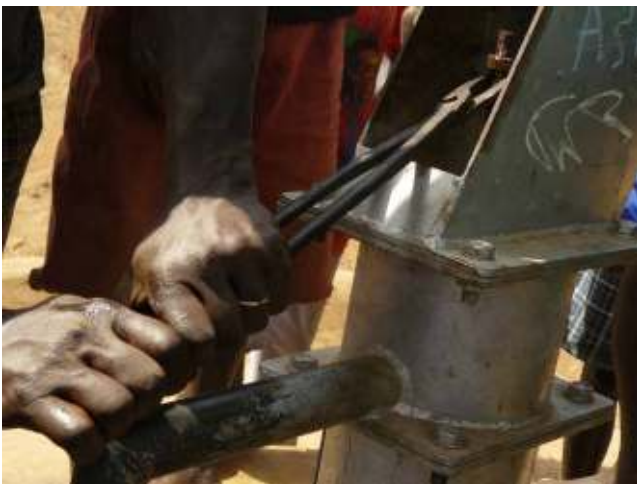
Fixing of handpump
