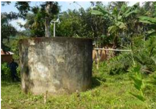
Previous situation: Wugbadu tank
