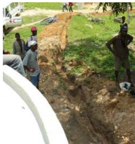
Kwangor – new pipelines
