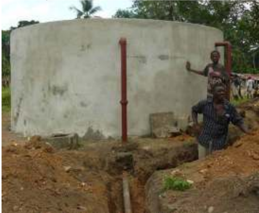
Kwangor gravity tank
