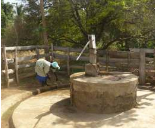
Rehabilitation with India Mark II handpump
