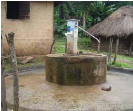
Rehabilitation with India Mark II handpump
