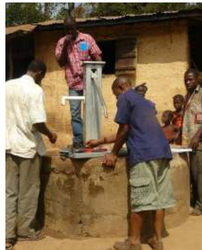
Installing new handpump
