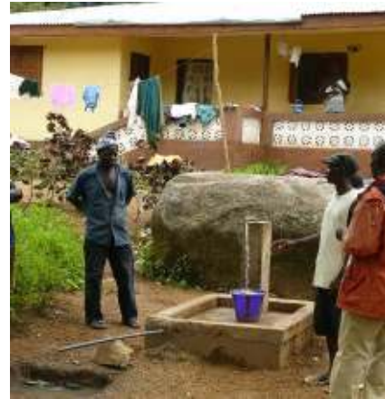
One Mile new standpost
